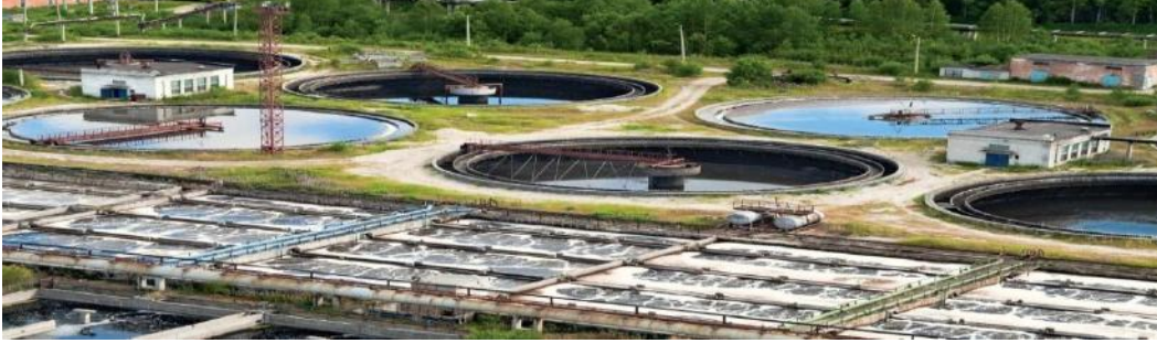
Image 2: Water Treatment Plant
